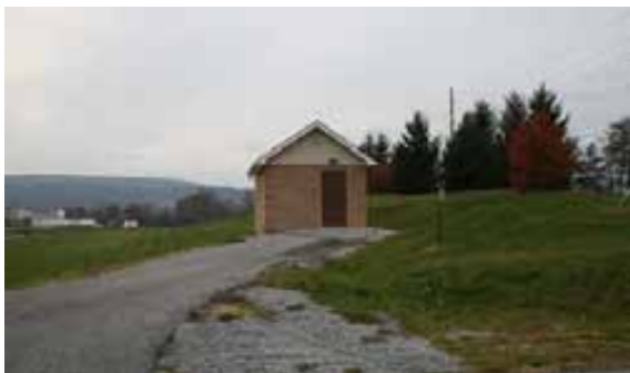
Photograph 2 Existing well house at the intersection of PA 103 and Arrowhead Way
