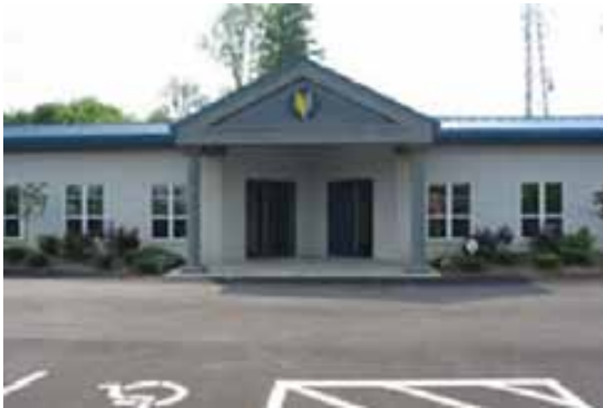
Photograph 16: Abele Business Park (photographic provided by Beynon & Company, Inc.)
