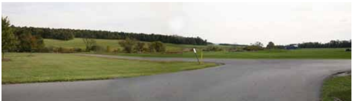
Photograph 9: Phase One "pad ready" parcels along Lenape Drive
